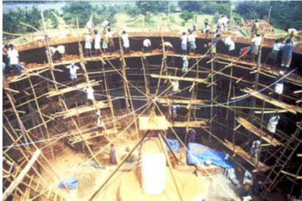
Up to 25 masons and 75 workers working on scaffolding
